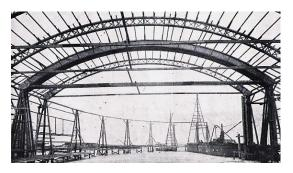
Figure 6: Two-hinge arch with tie (Tuchscherer 1918)
