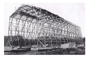
Figure 3: Airship hangar under construction (Estate Tuchscherer)
