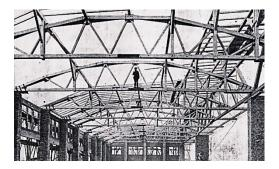
Figure 5: Parabolic truss (Tuchscherer 1918)
