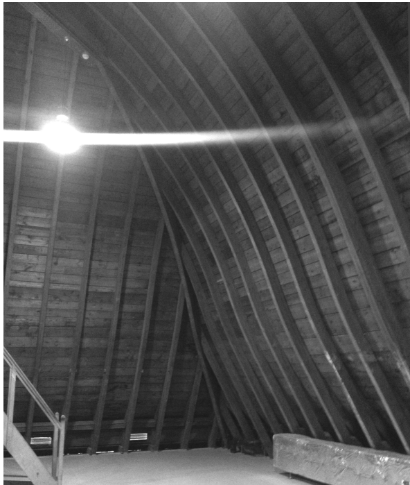
Figure 4: (a) Roof Structure of the Cupola of the University of Zurich (1911) and (b) platform roof in Interlaken (1921) (Chopard 1925)
