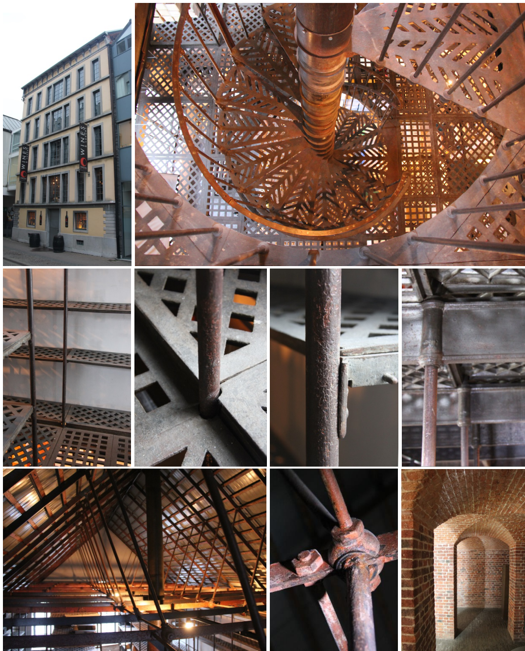
Figure 1: The Archive Depot in Antwerp, designed in 1851, consists of an iron stack. 1: Front façade - 2: Central iron staircase connecting the five floors of the stack - 3: Iron bookcases and floor grids - 4: Connection between floor grid and lower bookshelves - 5: The cast iron bookshelves are supported via bars which are screwed into the wrought iron column - 6: The wrought iron column fits within the cast iron beam - 7: The roof consists of slender wrought iron bars - 8: The columns are connected to the lowest bar of the roof - 9: The ground level which houses the heater is covered with brick vaults.
