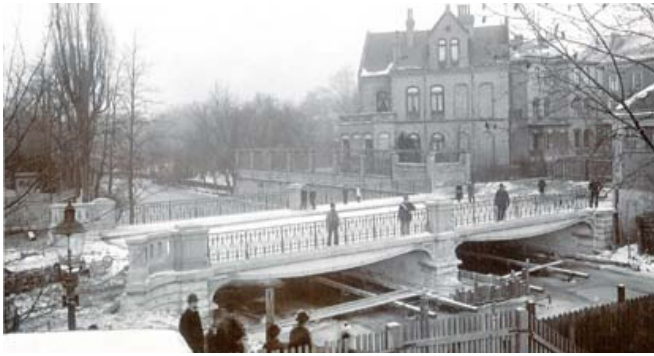
14 Ferdinand-Brücke, Braunschweig, 1901 [TB BS 1.03.11]
